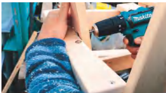
... while the impact driver made 90mm screws bump into softwood with ease
